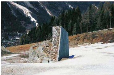
FIG.: Protecting wall in armed concrete at Taconnaz
